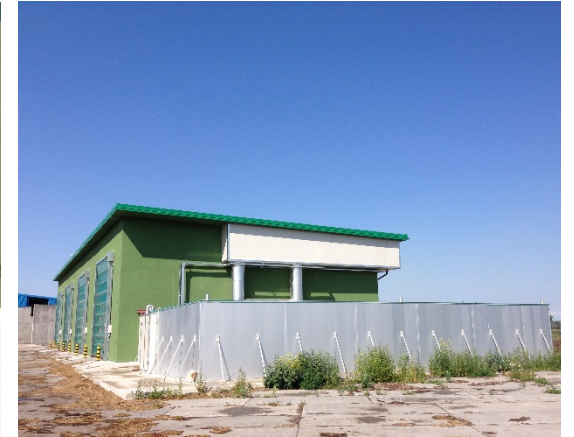
4. BIOFILTRO TO TREAT PROCESS AIR
